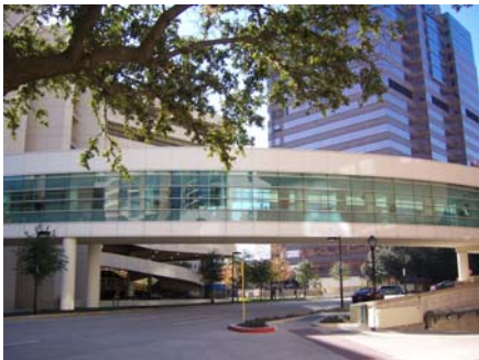
St. Luke's Episcopal Hospital – Garage No. 2 – skywalk
