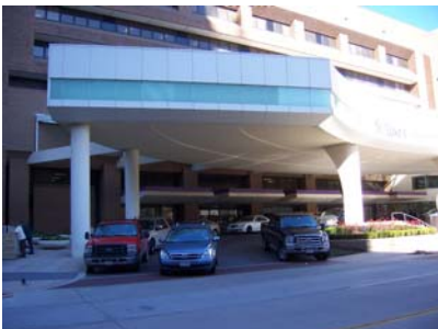
St. Luke's Episcopal Hospital drop-off driveway
