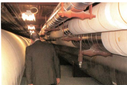
Skywalk with utilities
