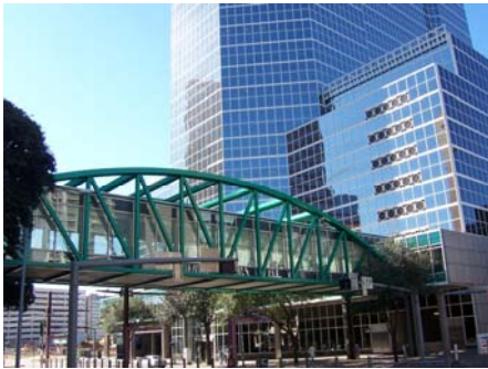
St. Luke's Episcopal Hospital – Fannin Street skywalk
