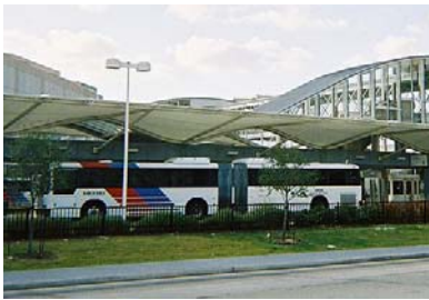
METRO Transit Center
